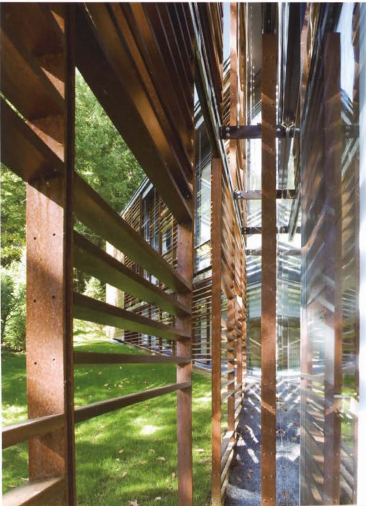
This page, above: Gatehouse and guest houses are situated throughout 21 acre site. Family house and recreation building are located along the lake on southeast side. This page, below: Close-up of wood screen and glass facade. Wood screens modulate privacy and scale the facade. They also control the amount of sunlight and soften interior light. Opposite: View of sunken courtyard of family house.
